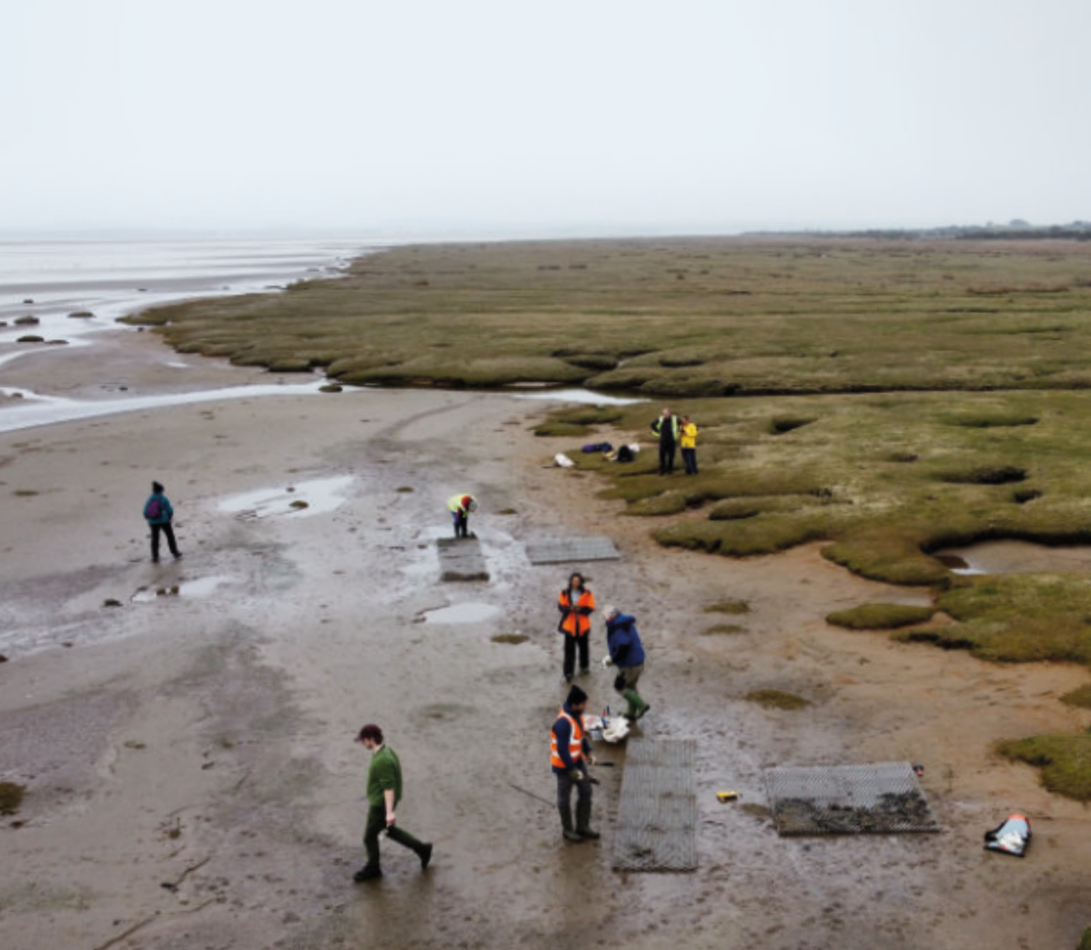
Installing BESE-elements® at RSPB Campfield Marsh
