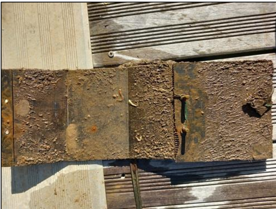
Photo 5 – Panel 1 Opened Out
