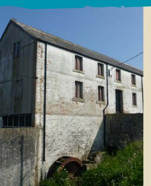
The building known as Wylie's Mill on Mill Street, Drummore, was still in use in the 1970s. However, despite the name, it was apparently always a grain store rather than a mill: the cast-iron water-wheel, visible at the north-west facing elevation, is thought to have powered a grain bruiser and a grain dresser. The floors and cast iron uprights are said to have been reused from a building constructed for the Glasgow Exhibition of 1901.
