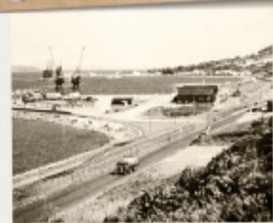
SOUTH DEEP WHARF AND MILITARY RAILWAY, CAIRNRYAN
