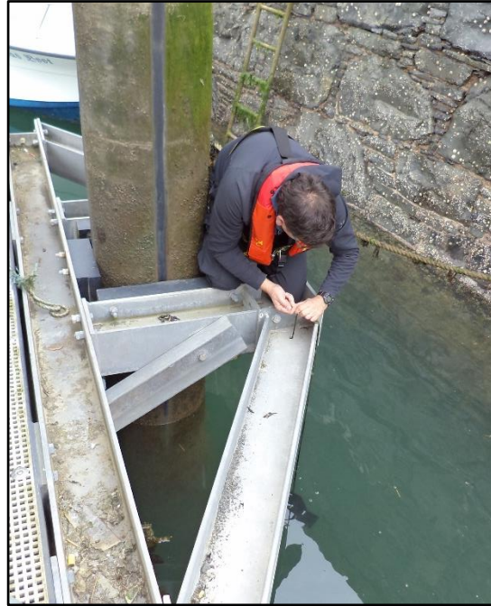
Photo 2 - Attaching panels
