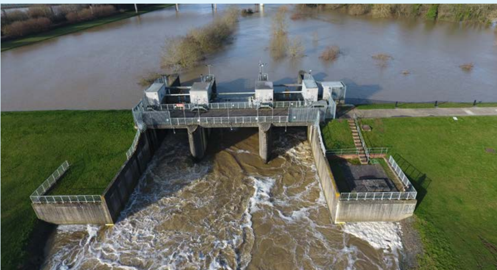
Figure 21: Leigh Flood Storage Area in operation, Kent.
