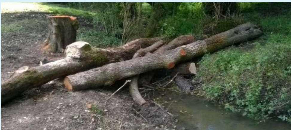
Figure 15: Leaky dam; one of the measures used in the Stroud rural sustainable drainage project.
