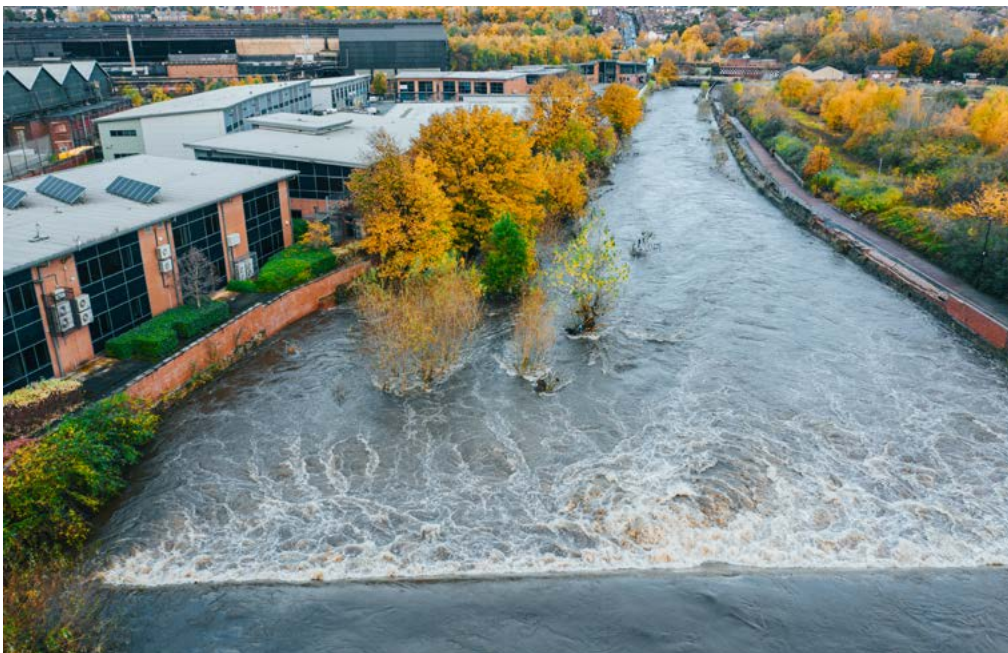
Figure 5: Damage caused by the River Don, Sheffield, Yorkshire, UK bursting its banks in the November Flood near Meadowhall, 2019.
