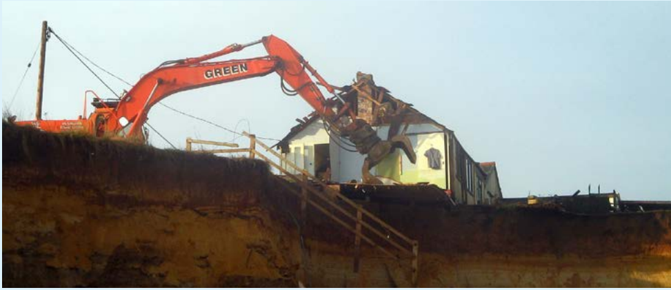
Figure 13: A property at risk of coastal erosion being demolished (image courtesy of North Norfolk District Council).
