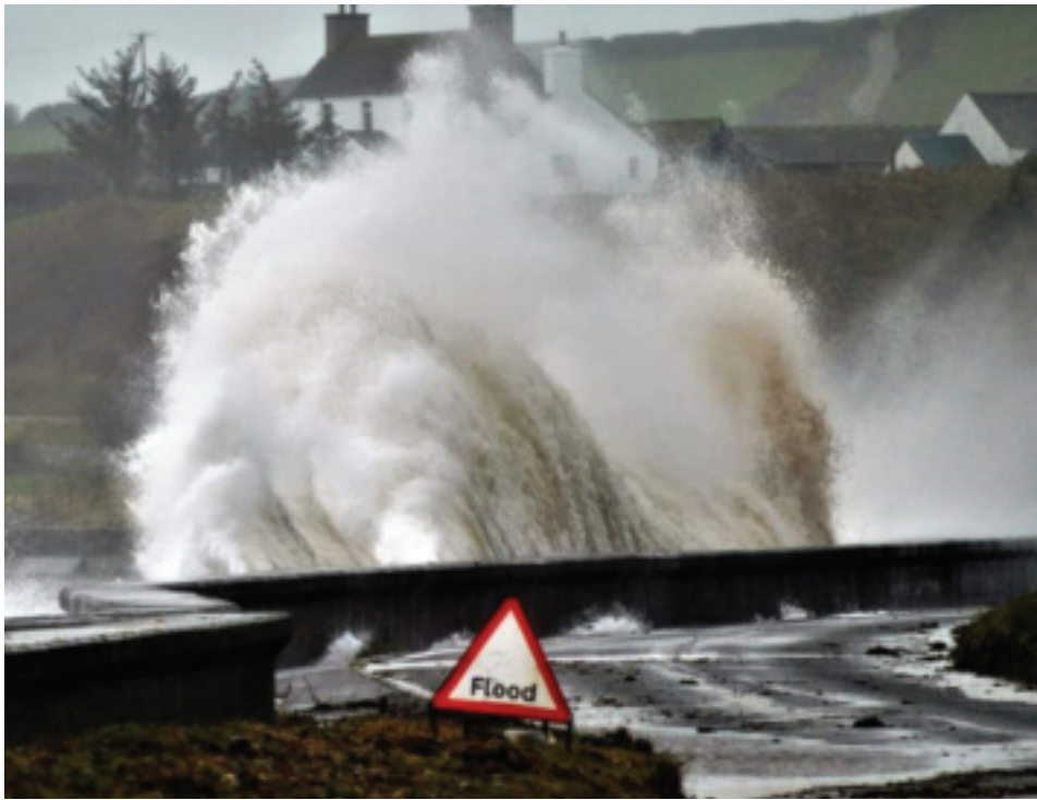
Wave over-topping on the coast
