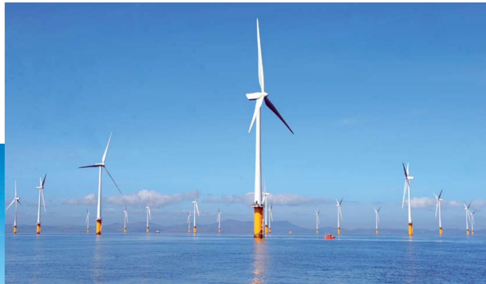
Robin Rigg Offshore Wind Farm
