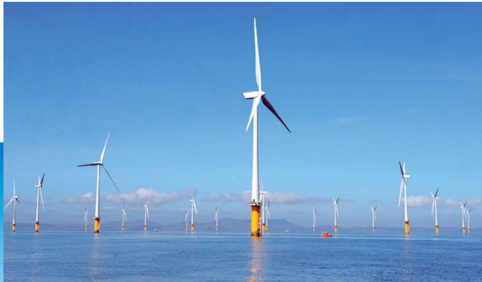
Robin Rigg Offshore Wind Farm
