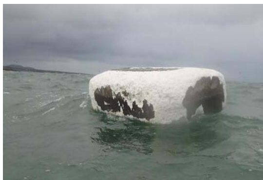
Fig 3. Remains of floating pontoon with surface resin (Photo credit: Ashley Williams)
